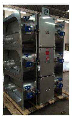
CTC Model B1-212-3x2-RCD22x48 (above), with round or oval dampers which are difficult to insulate and ship without risk of damage. Best to insulate in the field (after making duct connections) using a soft-wrap, insulation, as pictured below on a B2-series housing w/dampers.
