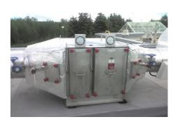
Condensation is going to be a problem for any Bag-in/Bag-out (BIBO) Filter equipment located outdoors, particularly in lower temperatures and in colder climates. Warm and humid building air will migrate upwards (even when the fans are off) through the exhaust duct and into the steel filter box where it will condense out when it hits the cold stainless-steel.
