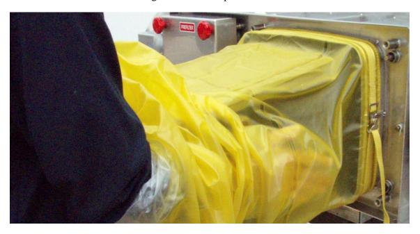
6. If using a cable tie, tightly twist a 10"-12" section, tie off each end, and cut in the middle. Use duct tape to securely tape each cut end. After isolating the contaminated filter, remove the safety strap and move the left over bag stub to the first rib of the bagging collar. This allows the new bag to cover the old bag stub while keeping the contaminated area secure.
