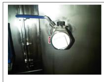
The standard decontamination port supplied with CTC filter housings is the 1.25" partial-bore ball valve. This T304 stainlesssteel ball valve has a 0.75" opening, more than sufficient to permit connection to a Certek™ paraformaldehyde generator unit. This is the industry-standard decon unit used by Canadian contractors for decontamination of bio-safety cabinets and similar enclosures using paraformaldehyde gas.
