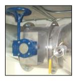
**DAMPERS:** Bubble-tight dampers can be provided on either or both sides of the housing to provide leak-free isolation. Dampers are available with manual, pneumatic or electric actuators. (*Left*)
