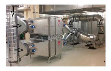
Bag-In/Bag-Out (BIBO) Housings feature continuous seam-welded stainless-steel construction. Housings are built to ASME N509 Nuclear Standard and every housing is pressure-decay (leak) tested to ASME N510 Std. Every housing is tested to ensure zero leakage at a minimum of 10"wg. As well, the filter clamping mechanism assures that HEPA filters can be certified to true 99.97% efficiency performance on 0.3 micron and larger particles.
