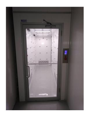
Standard construction for air showers is epoxy-painted steel, with anodized-aluminum doors and PLC controller with push-button LED controller adjacent to the entry door.
