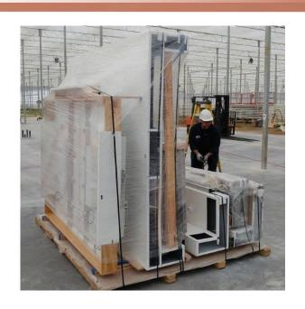
Larger units, and units being installed in tight spaces, have to be broken-down at the factory (after complete assembly and testing) for reassembly at the site. This requires a conscientious contractor to ensure a proper, airtight installation. Showers that are going to be site assem-
