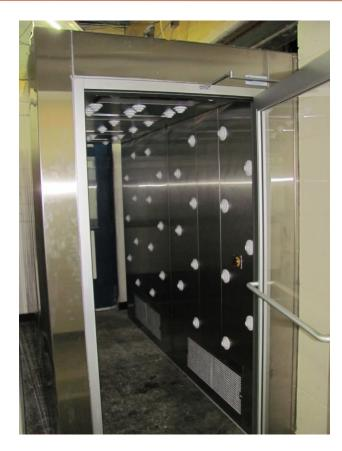
When high personnel thru-put is required, the best option is an air-tunnel. When an Ontario food processor needed an air shower installed to meet corporate and cGMP requirements, they decided to purchase a 3x10 air tunnel. The motion activated fans allow a continuous stream of personnel into the cleanroom, eliminating the need for door interlocks. Side mounted filters and fans were required due to low headroom in the changeroom corridor.
