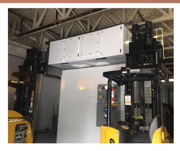
For large, custom showers like the one pictured here, site assembly by an experienced installer is mandatory. This model AS8109 (8'x10'x9' ID) shower with two high-speed roll-up doors arrived at the site in (3) large crates, weighing approx. \_\_\_\_\_ -lbs. Installing the two top-mounted filter-fan cabinets required a lot of finesse, given only a few inches of clearance to the trusses above.
