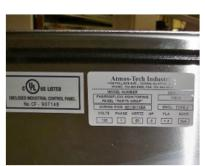
Atmos-Tech air shower electrical panels are designed and built at their in-house UL508A certified panel shop. UL508A certification means they can apply the c-UL mark on all their electrical panels (see pic at bottom left).
