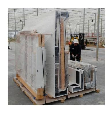
Larger units, and units being installed in tight spaces, need to be broken-down at the factory (after complete assembly and testing) for reassembly at the site. This requires a conscientious contractor to ensure a proper, airtight installation. Showers that are going to be site assembled should be installed immediately after floors are finished.
